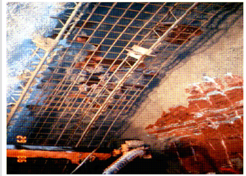
passive support for span area inside the tunnel
