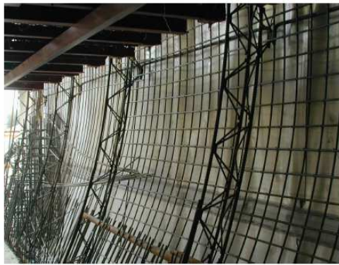
Providing support for steel fabric to bear the loading of cement in Final Lining
