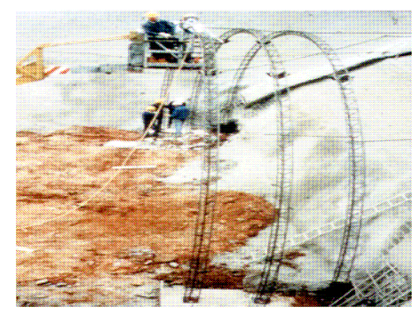
Tunnel portal support before excavating
